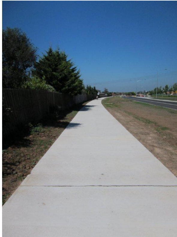
Figure 3. E-Crete Footpath (Calder Freeway Interchange)
