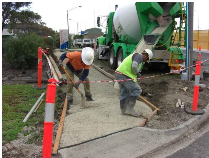
Figure 2. E-Crete Placement (Port Melbourne)
